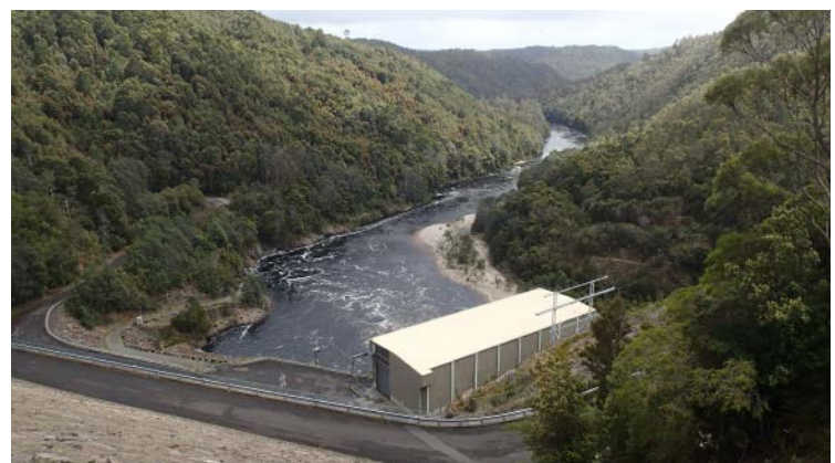
Middle: Lake Pieman at the dam wall on a very windy day. Above: Looking downstream over the building that houses the generators. Photos: Greg Martin
