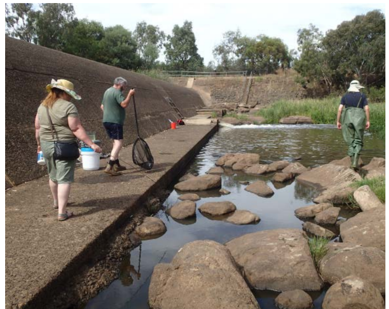
The Southern Water Diversion Weir wall. Photo: Greg Martin.
