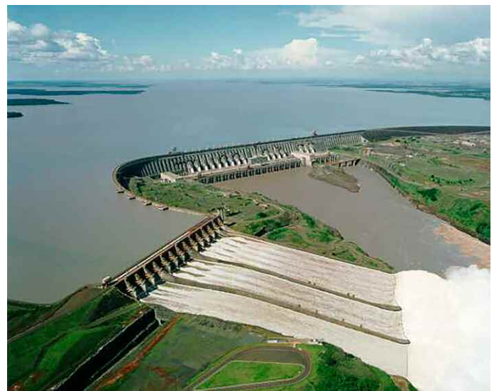
The massive Itaipu dam, located at the Brazilian-Paraguayan border and not far from the Argentinian border, supplies approximately one-fifth of Brazil's energy. The water behind the dam took only two weeks, due to heavy rain, to rise 100 meters filling the reservoir. Each year ITAPU generates 75 TWh of electricity and avoids 67.5 million tons of carbon dioxide emissions - compared to coal power plants. Source: Wikipedia
